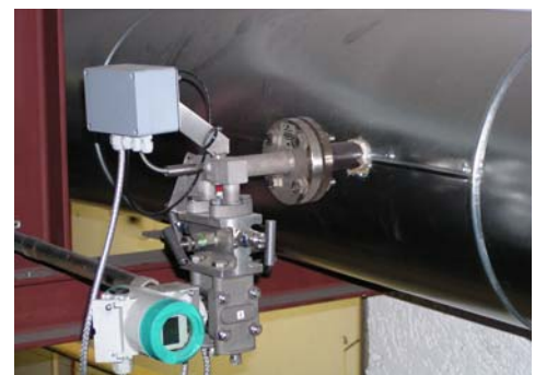
Figure 3 : deltaflow for steam with integrated PT100, 3-way-manifold, mounted transmitter and connection box for cables
