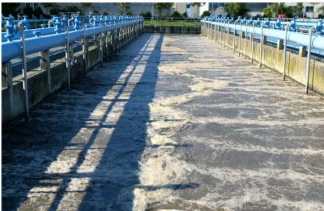
Insufficient oxygen supply results in incomplete decomposition of harmful substances and thus insufficient cleaning performance. In the worst case, statutory limit values might be exceeded.
