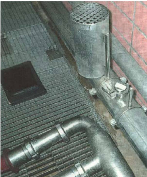
Illus. 1: pH measurement point with Durafet II sensor in casing
